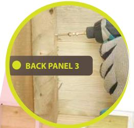
Screw sides to secure against the previous back panels post as shown here.
